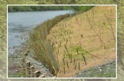
Bioengineering corresponds to the techniques and strategies using plants for soil erosion control and management. It aims at achieving objectives of restoration, rehabilitation or reaffectation of eroded areas.
